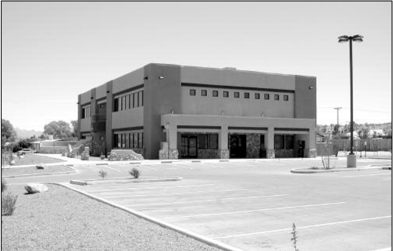
Southeastern Arizona Behavioral Health Service (SEABHS) new administration building. Photo: John and Jeanie Mangold
