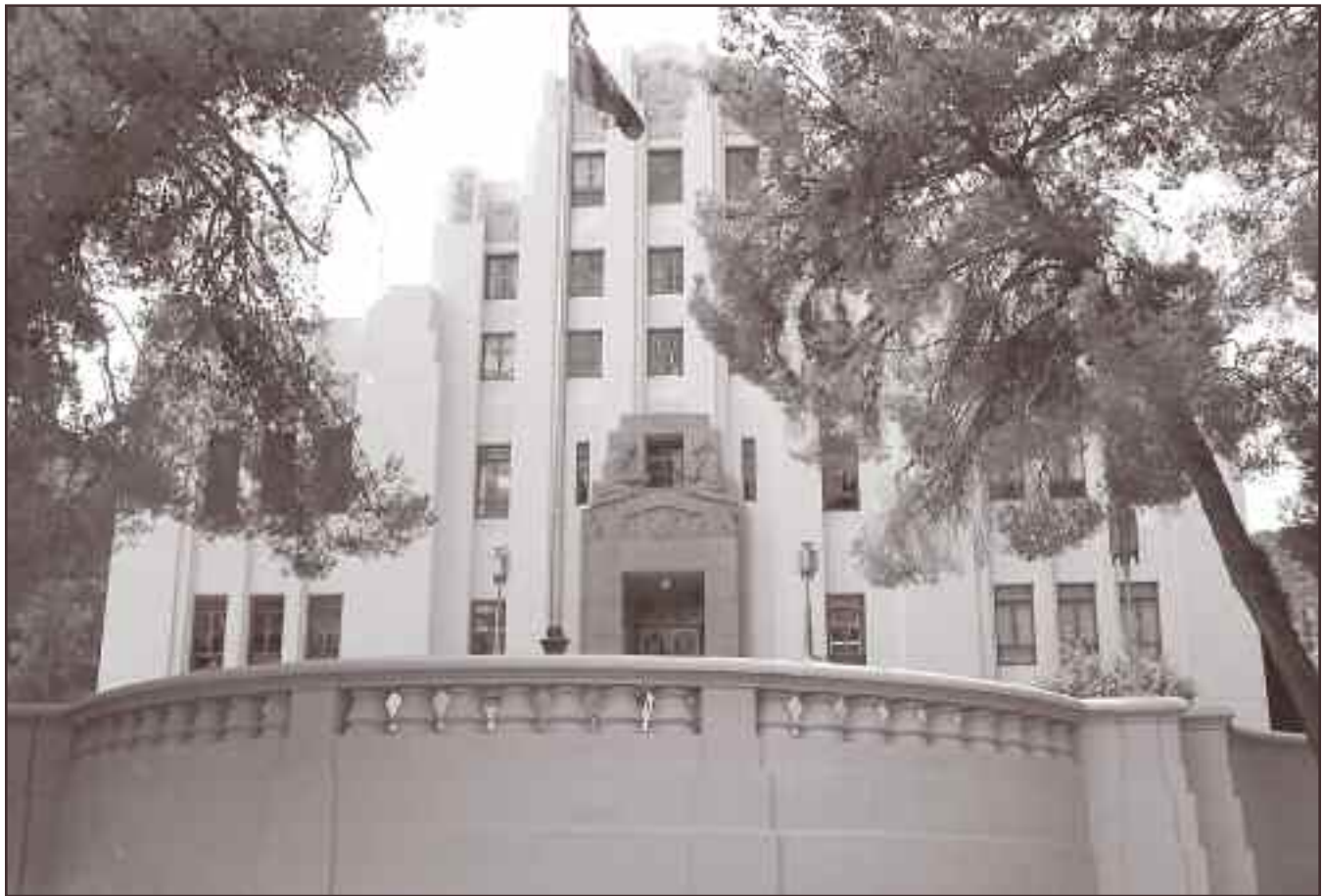
Cochise County Courthouse located in historic Bisbee.
