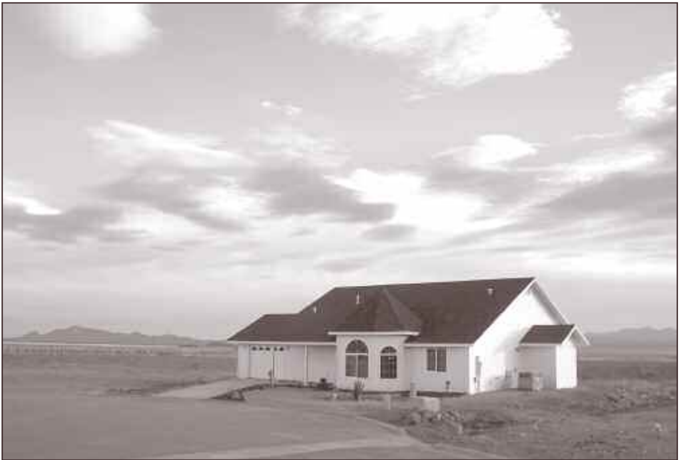
Construction on the homestead development project in the San Jose district of Bisbee.
