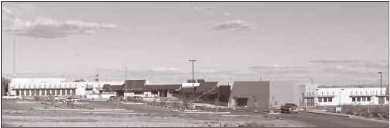
A panoramic view of the new Cochise County Complex.
