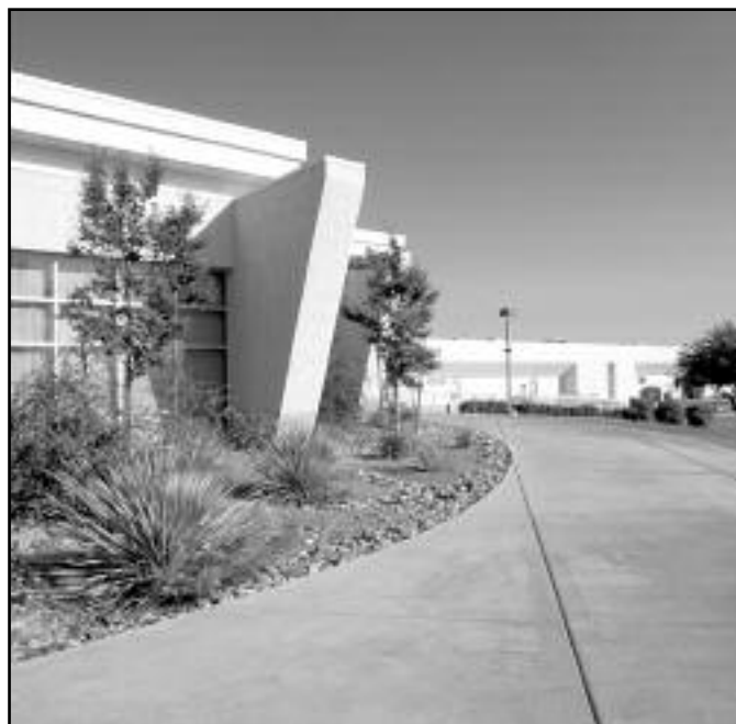
Walkway outside the Sierra Vista Cochise College Campus library.
