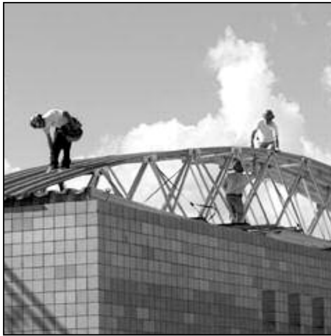
Commercial Construction. Photo: Justin Levesque-Herald/Review
