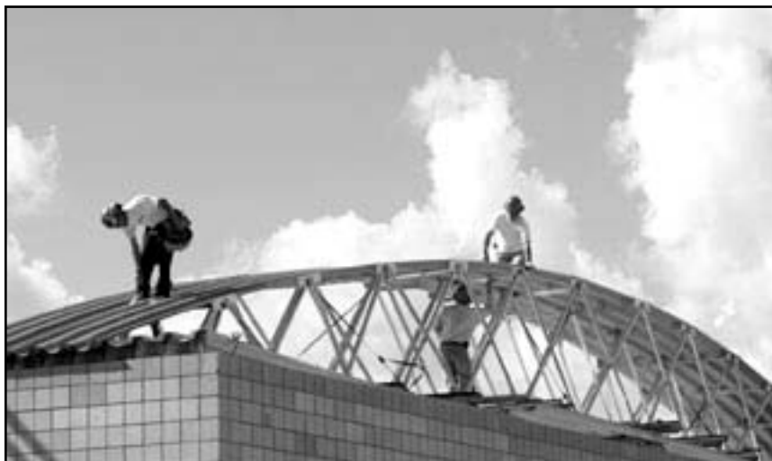
Commercial Construction. Photo: Justin Levesque-Herald/Review.
