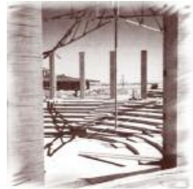
Cochise College under construction
